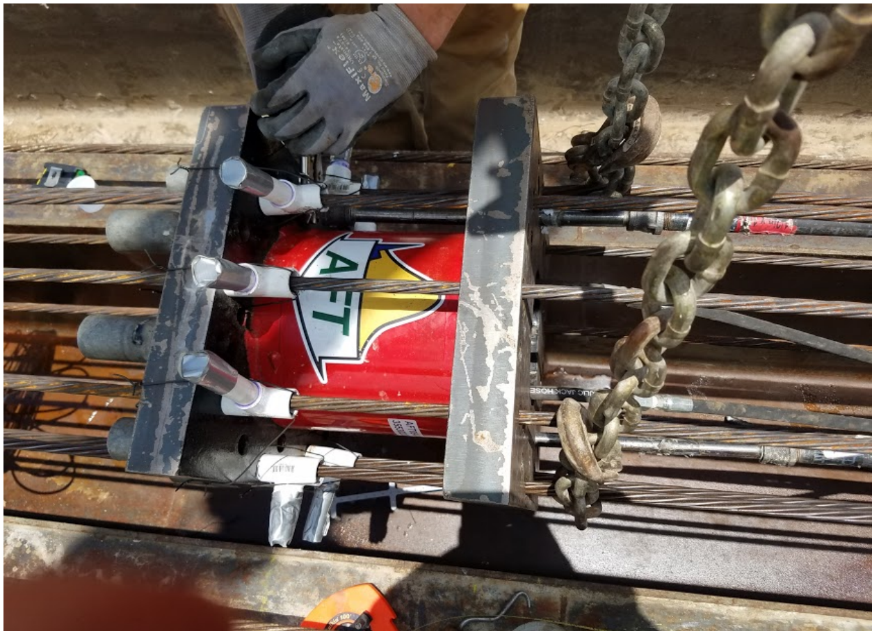
Figure 4.4-4 Photo of the AFT cell installed in the pre-stressed concrete pile.
