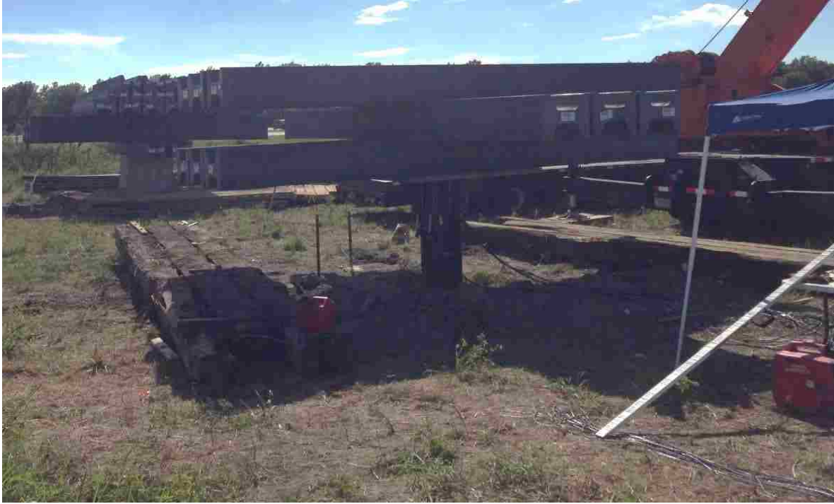
Figure 4.4-8 Photo of the loading configuration completed.
